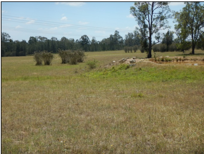
Figure 6: Existing dam on site
